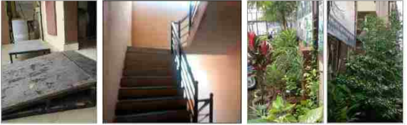
Provision of Ramp, staircase with handrails and Garden spaces in the premise
