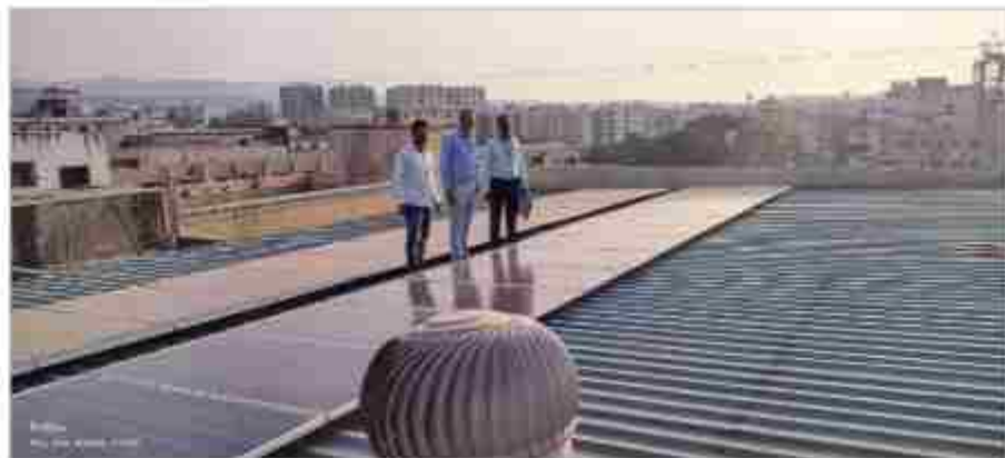
Energy efficient fan and solar roof top
