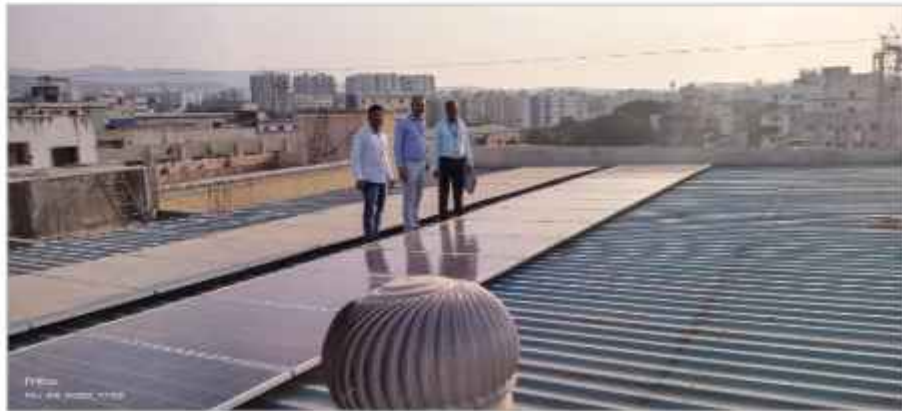
Energy efficient fan and solar roof top
