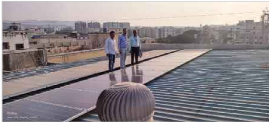
Energy efficient fan and solar roof top
